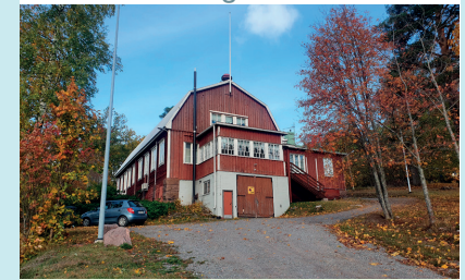
Seutula volunteer fire brigade building, Vantaa
